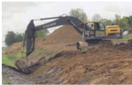
Parkway Construction I-69 and Pennyriple Interchange Job
