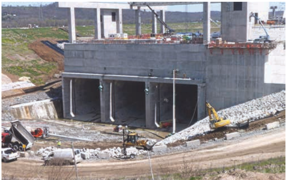
Working on Outlet on Meldahl Dam with Aquarius Marine
