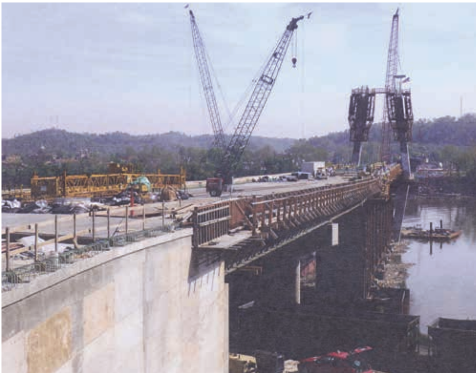
The Ironton Russell Bridge project continues to be on schedule.
